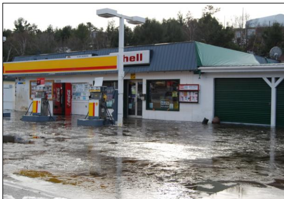
Flooding in Pointe au Baril, January 2008
